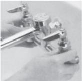
STEP 2: Next, remove the old control valve body by unthreading the nut.
