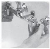
STEP 4: Then thread your new Zurn faucet body onto the AquaSpec adapter and tighten. (Discard supply arms supplied with new faucet.)
